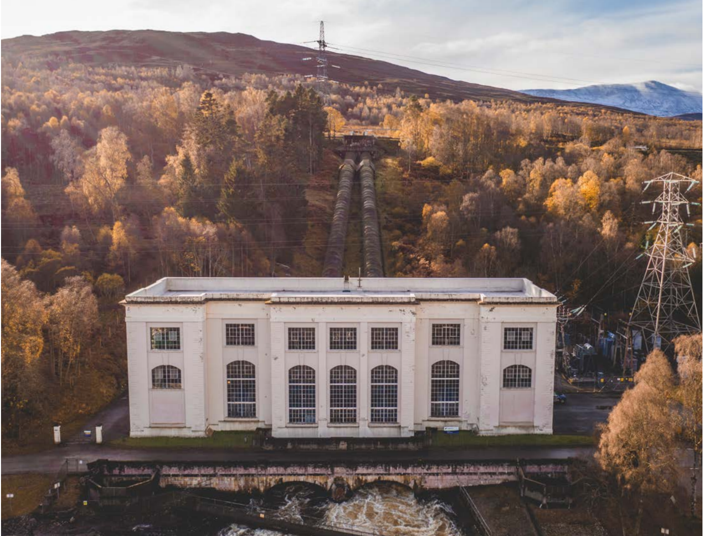
Tummel Bridge Power Station
